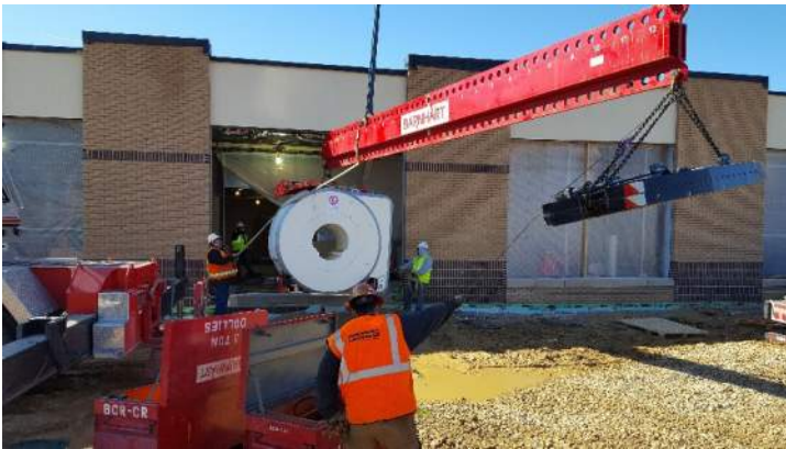
The MRI was moved into place through an exterior window and a crane using counter weights as shown in the photo on the left. The MRI now sits in its final room which is nearly ready for use! The photo on the right is the view of the machine from the control room.
